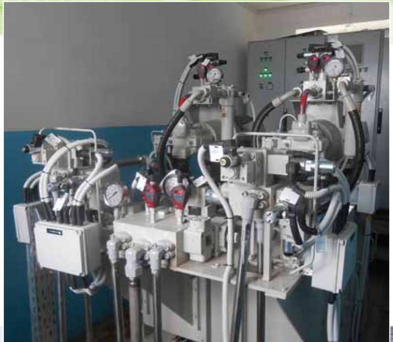
Double hooked gates control block
