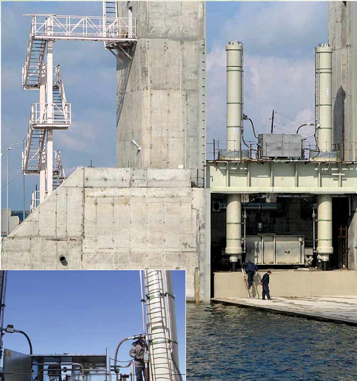
Control block for synchronization of cylinders operation on the left and right side of the gate
