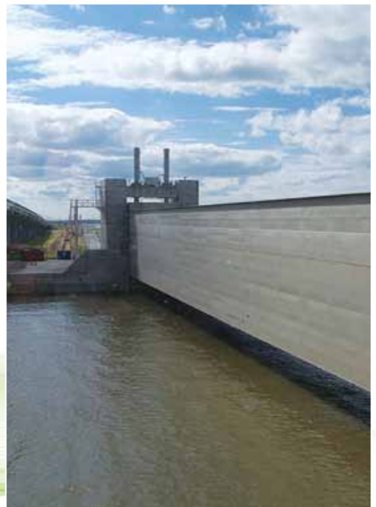
Flat gate in overhaul position
