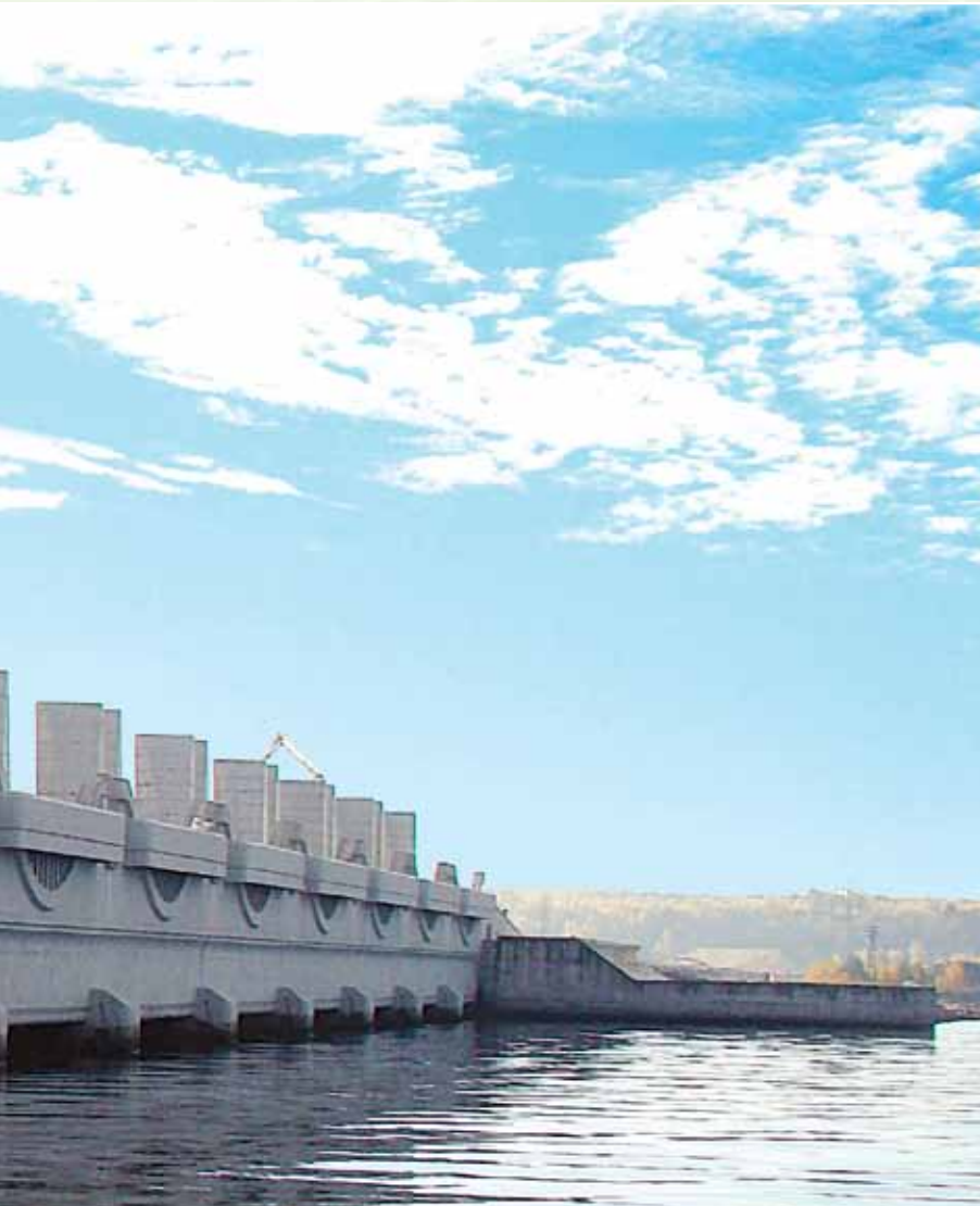
Water discharge facilities V1-V6
