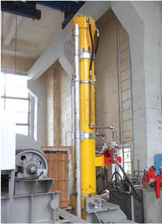
Electro-hydraulic system for handling gates
