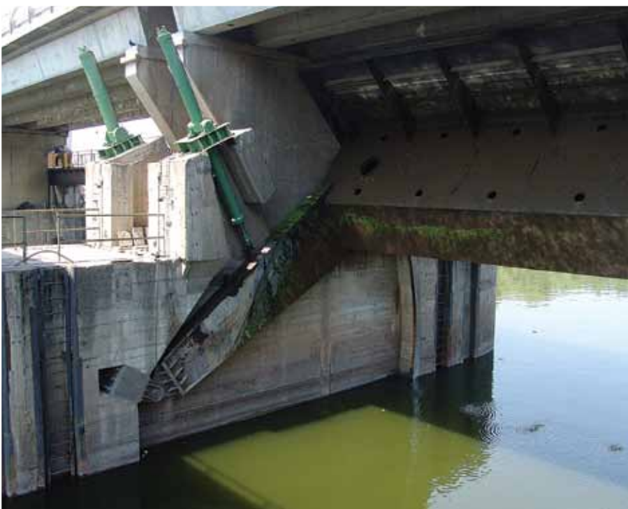
Floodgate Pančevo – segment gates cylinders
