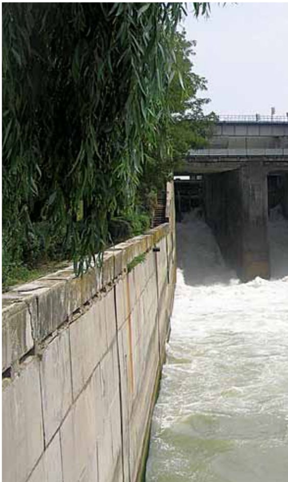
First and second passage of dam spillway field
