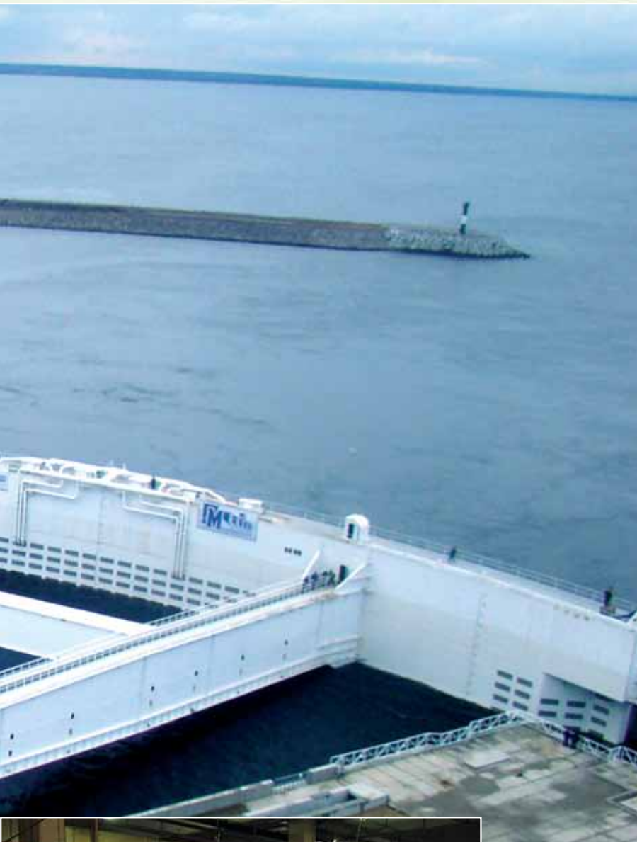
Complex of flood control structures of Saint Petersburg – sectoral gate – bataport
