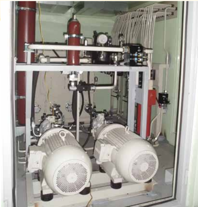
Metallurgical plant Severstalj
