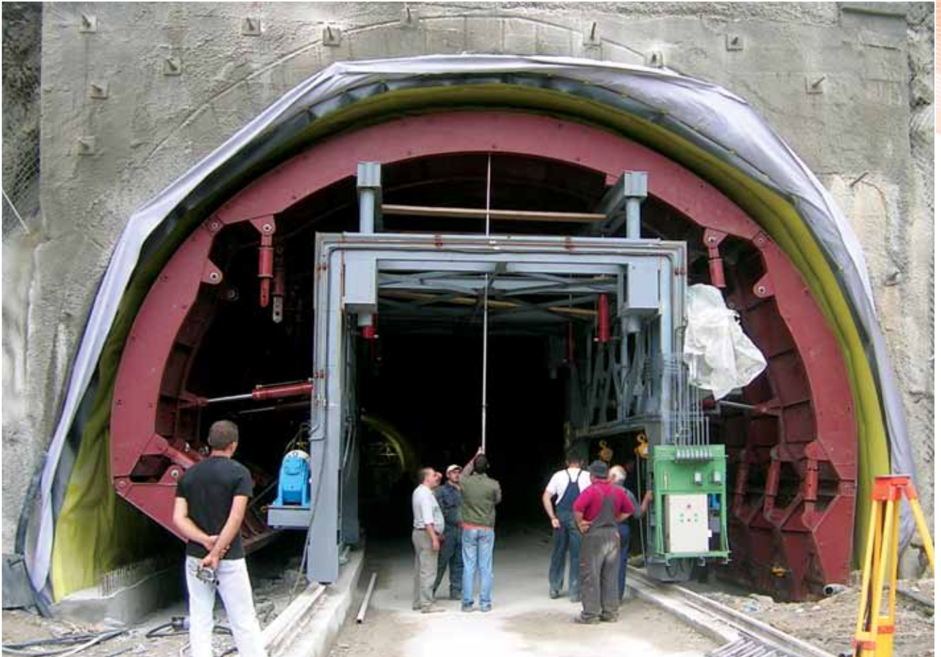
Hydraulic telescopic casing for concreting of tunnel
