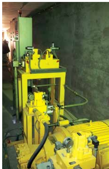
Quick closing gates hydraulic agregate
