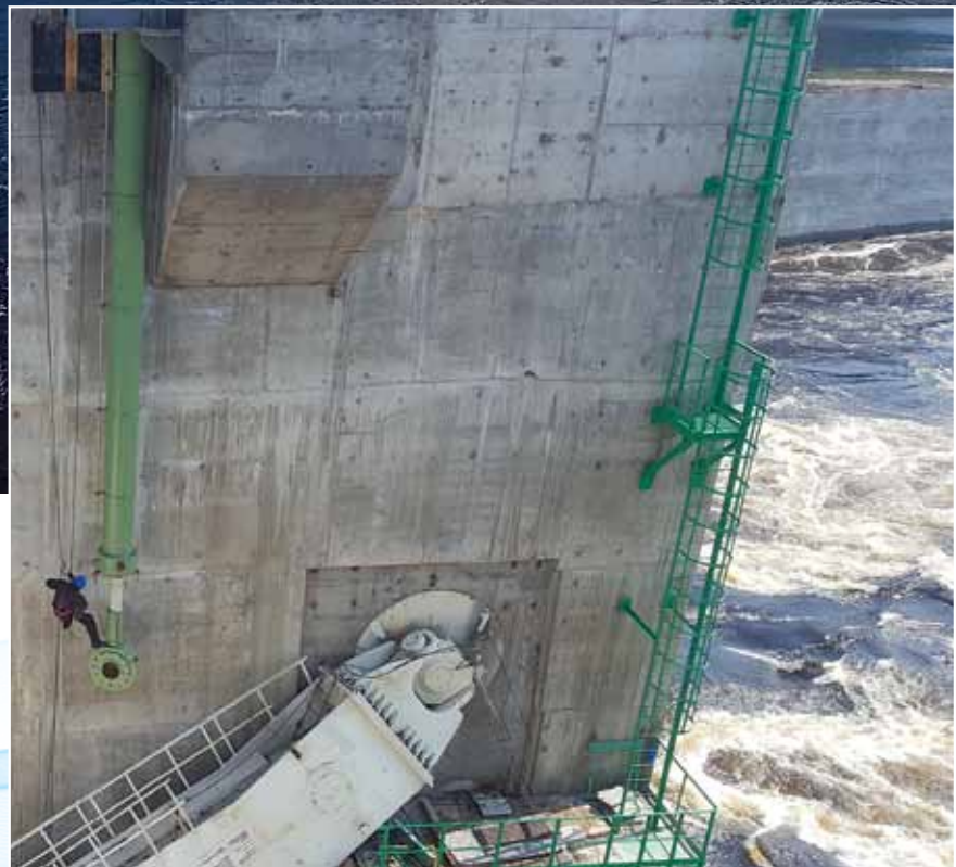
Segment gate cylinder
