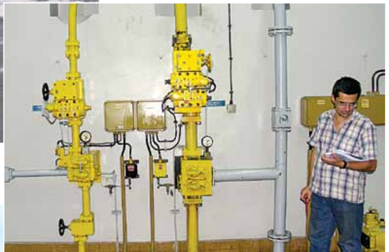
Djerdap 1 – Control blocks on ship lock middle head
