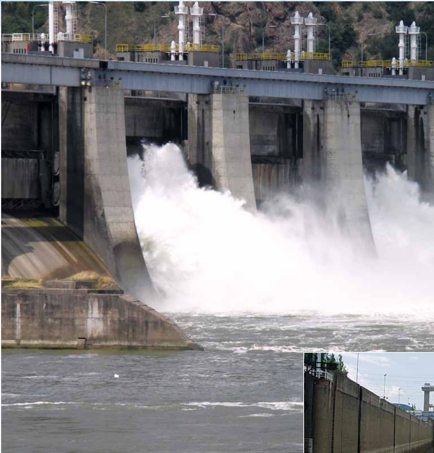
Dam spillways – hydraulic installations of double hooked gates
