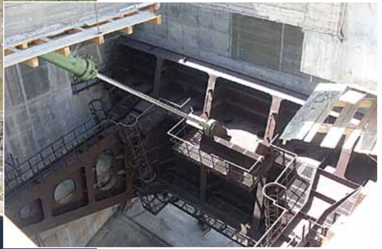
Spillway segment gate cylinder
