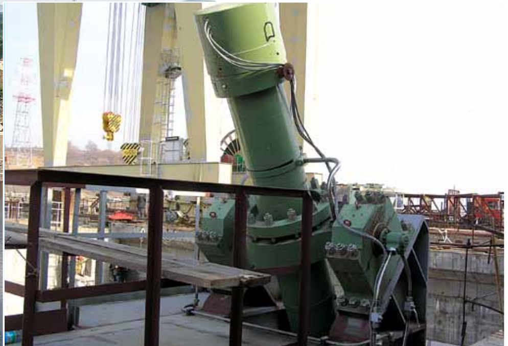
Segment gate cylinder with support
