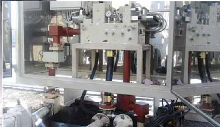
Djerdap 2 – Quick closing gate control block
