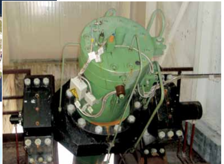
Spillway segment gate cylinder with hoisting trunnion and control manifold
